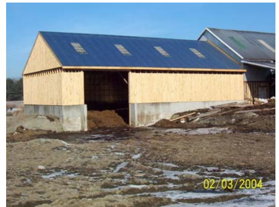
AFTER – the new walls and roof will lessen run-off
