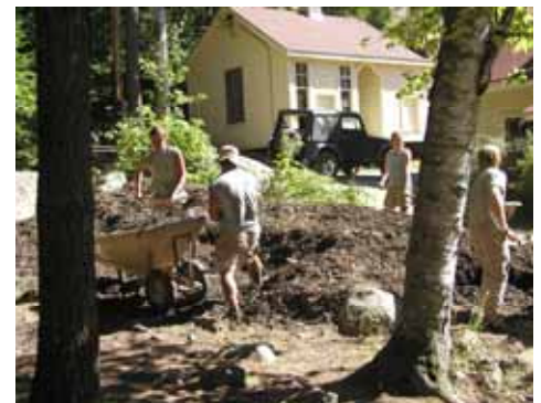
Spreading 48 yards of "Slope-Stabilizing" mulch at Pilgrim Lodge on Cobbossee.
