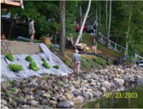
Installing buffer plantings & rip-rap on Maranacook Lake
