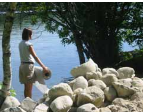
Laying geo-textile fabric before placing rock on Pleasant Pond.
